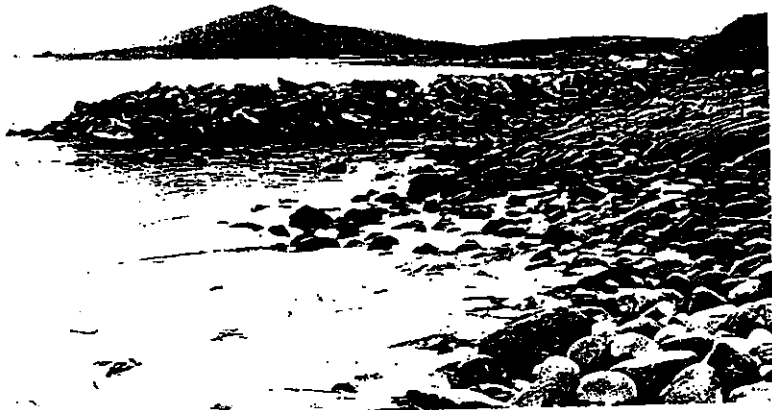
Figure 31 View of the Gabo Island Groin from the jetty.
